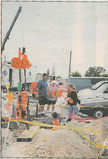
Photos above: Joyce Velitschkowski (at right in photo above) and a JTV crew prepare and calibrate equipment prior to a pipe inversion; JTV crew members conduct a lateral relining project.
