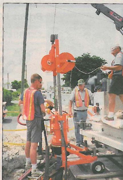
Photos above: Joyce Velitschkowski (at right in photo above) and a JTV crew prepare and calibrate equipment prior to a pipe inversion; JTV crew members conduct a lateral relining project.
