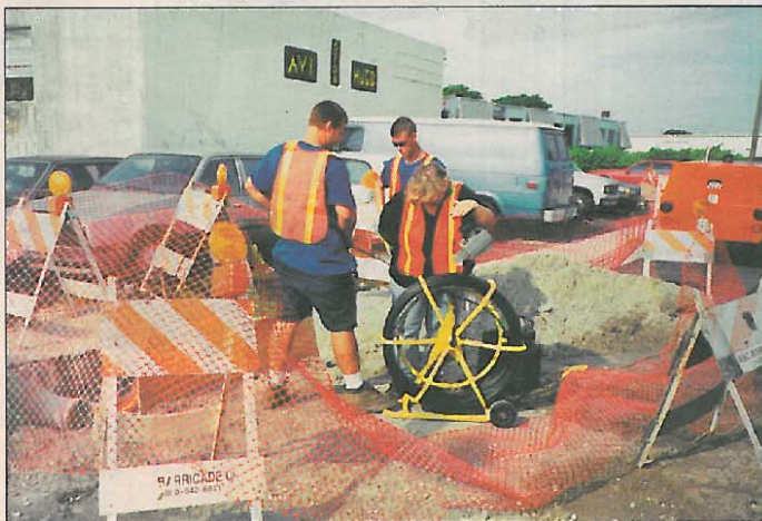
Top left: Joyce Taylor Velitschkowski, founder and owner of JTV, Inc., with one of her custom-built video inspection vehicles. Top right: JTV crew with a specially-equipped combination vehicle for large diameter pipe cleaning projects. Above left: Joyce and crew video inspect a lateral prior to lining. Above right: Joyce conducts a pipe survey using a Pearpoint mainline camera in conjunction with flexidata pipe survey reporting software.
