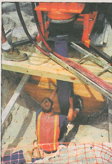
Photos above: Joyce Velitschkowski (at right in photo above) and a JTV crew prepare and calibrate equipment prior to a pipe inversion; JTV crew members conduct a lateral relining project.
